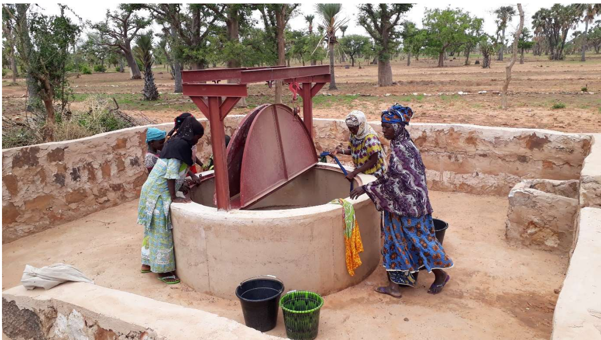
A modern cement well with a pulley system that allows 8 women to draw water at once.
