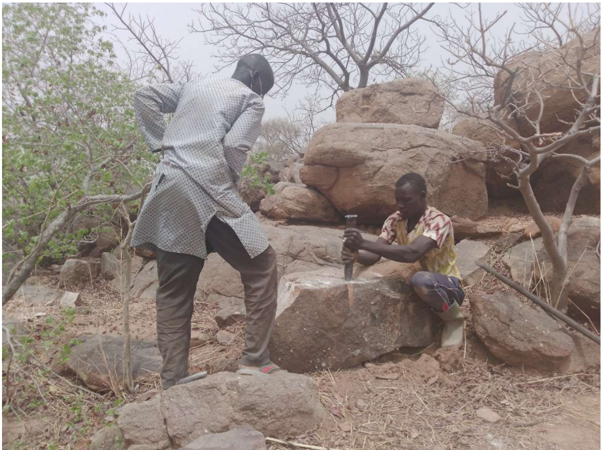
Breaking stones to build the stone lines
